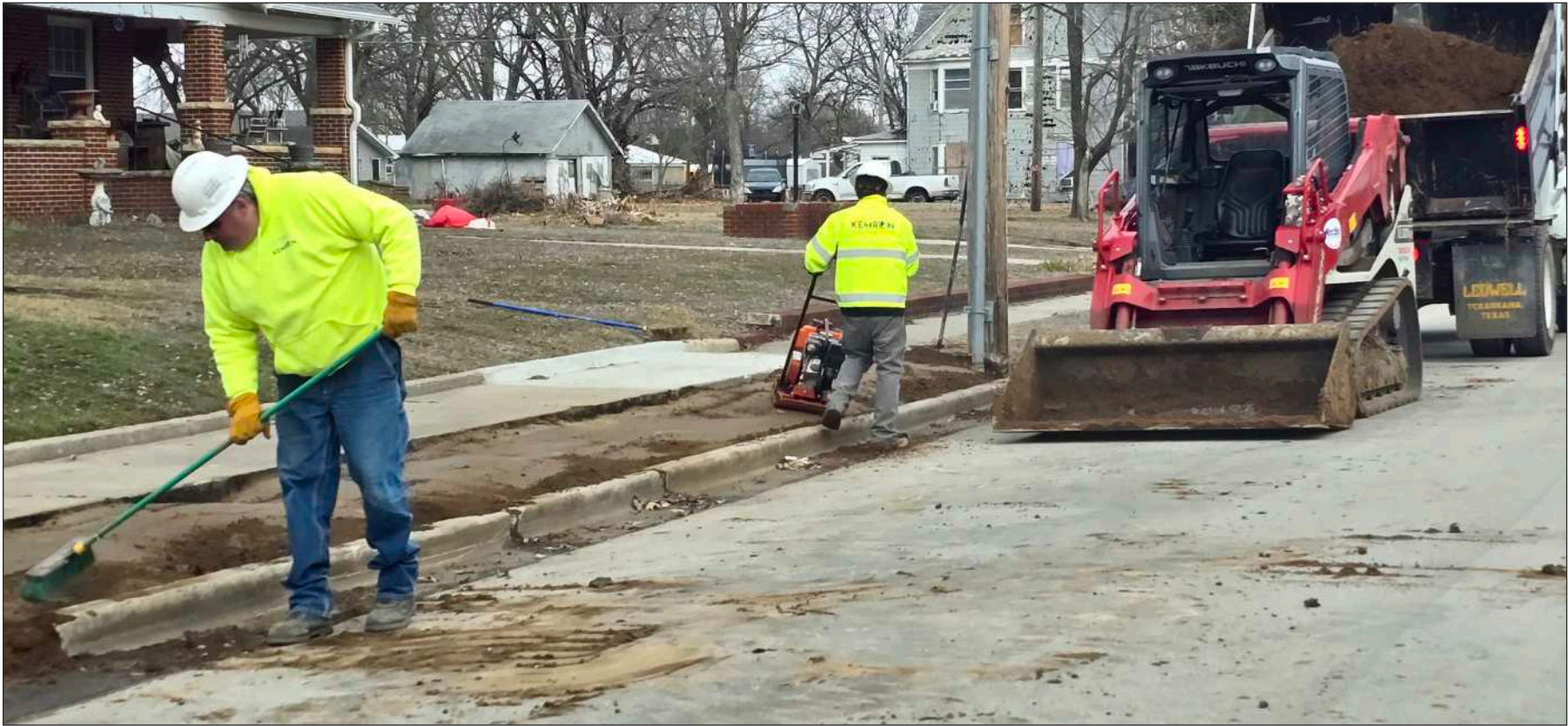
Crews from government contractor Kemron replace contaminated soil at an East Third Street property in Caney. ANDY TAYLOR / MONTGOMERY COUNTY CHRONICLE
