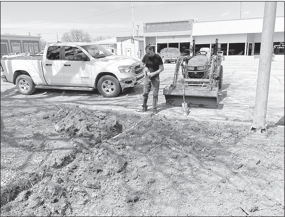
Grounds and Maintenance Supervisor Dave Schneider installs new sprinkler lines while restoring the outdated landscaping in front of the Hansen Museum to lush, green grass.
