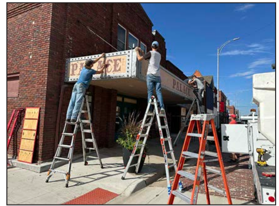
The workers at Mark's Custom Signs prepping the marquee for the new sign and lights
