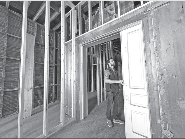
Frontier Development's Tyler Holloman opens original pocket doors that are part of a Broadway Lofts apartment.
