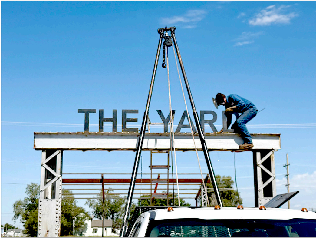
TOP PHOTO: COLE YOUNGER (left), with Tom's Machine & Welding Services of Plainville, and Adam Comeau (right), with Downtown Plainville, Inc., prepare to lift the final beam that will hold The Yard sign in downtown Plainville on Thursday, September 3. In the bottom photo, Cole welds "Yard" to the top beam. Each beam used for the project was salvaged from the historic Plainville water tower, which was dismantled earlier this year. (Photos Courtesy of Ashley Comeau)
